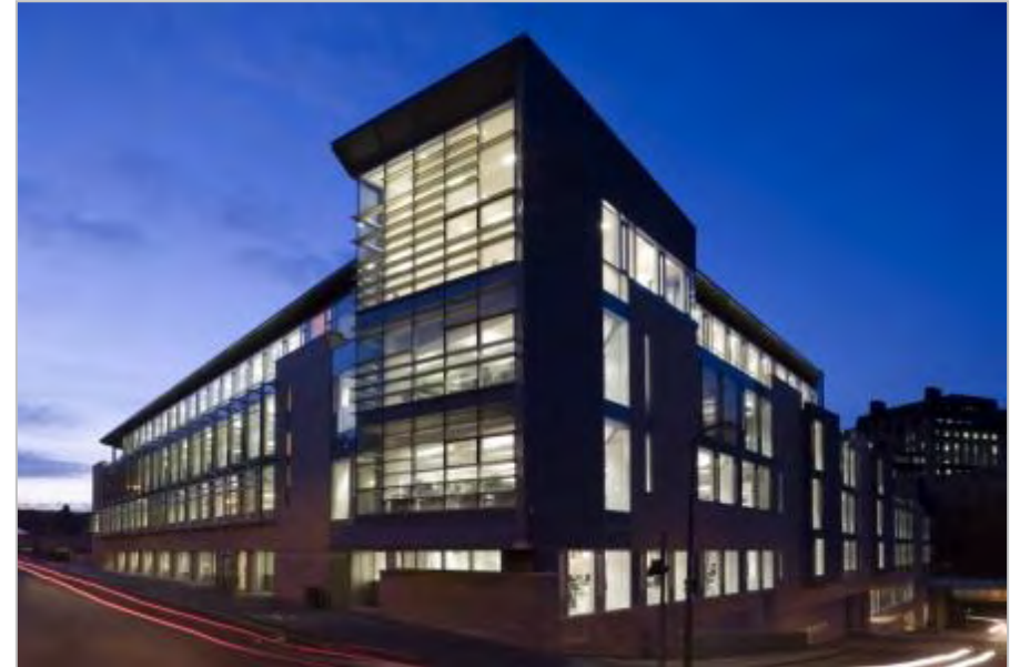
Council headquarters, East Market Street
